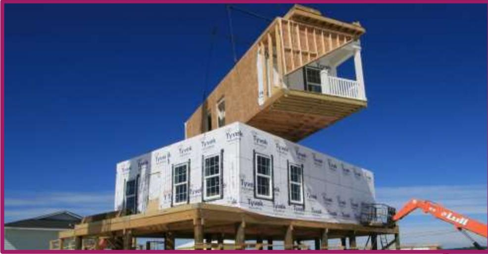
A modular home (or prefabricated home) is built in a factory to about 80-90% completion and then trucked over to the building site.
